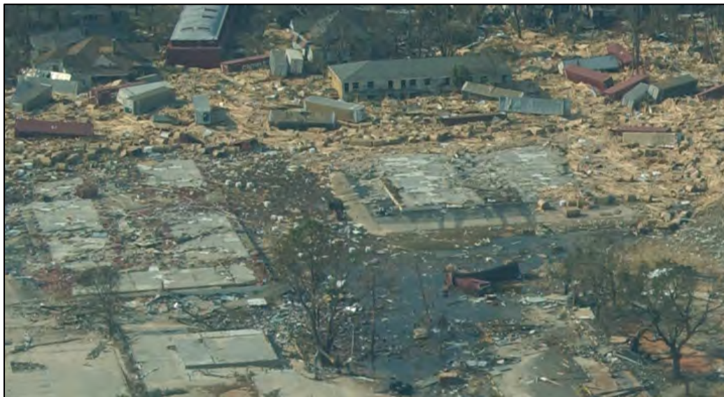
In this West Gulfport community located between Camp and Broad Avenue, freight trailers and barges coupled with the sight of concrete slabs from buildings and homes help show the magnitude of destruction. This photo was taken just a couple of days after Katrina came ashore – Hurricane Katrina 2005
